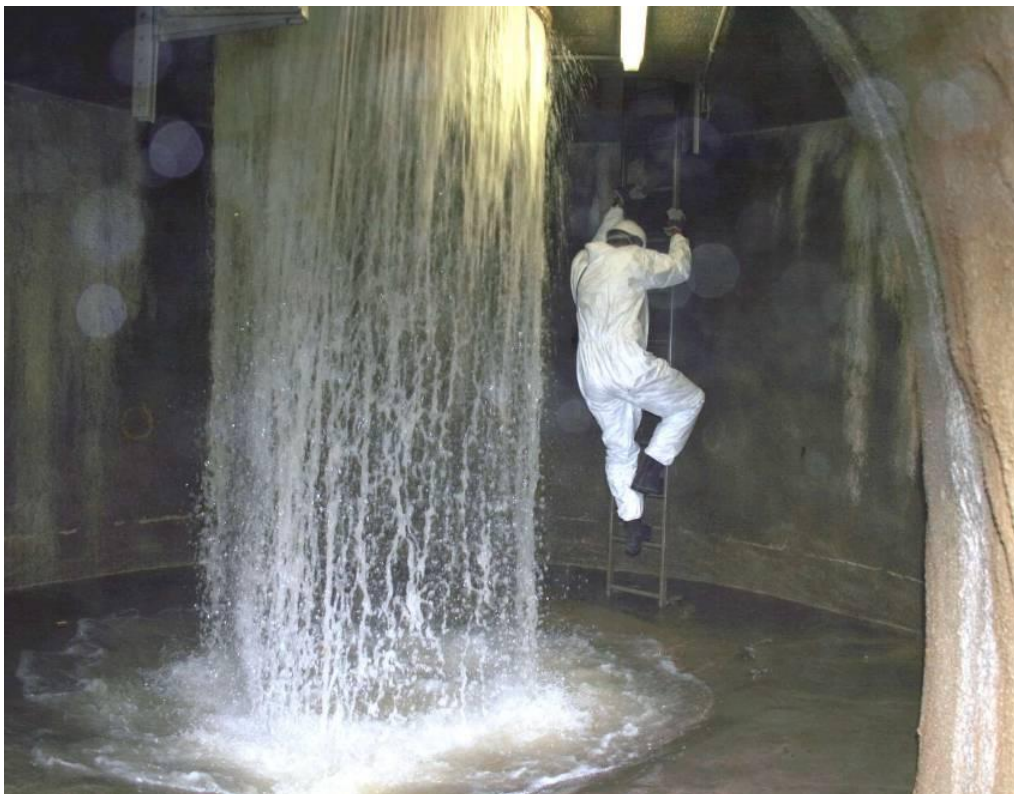
Fig. 8. Circular water jet falling down into the energy dissipation chamber of the Wiggen drop shaft during a minor rain event. The total drop head is 11.2 metres. (Photo: Hohl)
